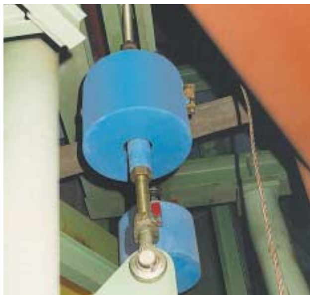
Spring hanger type 22 with clevis mounted.
