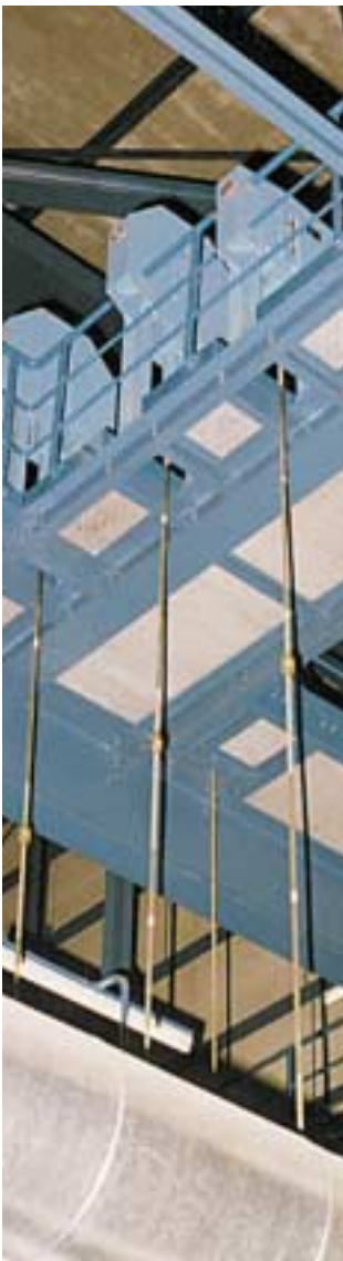
LISEGA constant hangers installed
